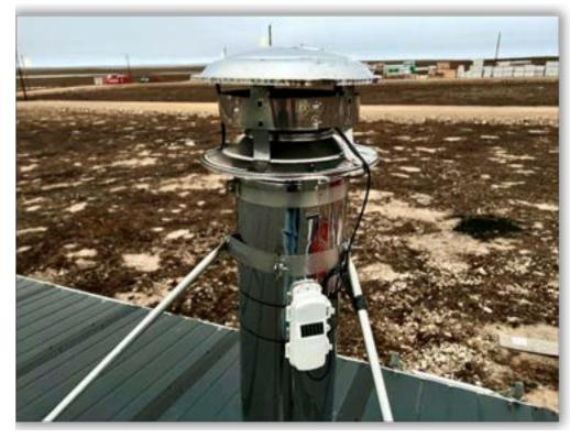
**Fig. 1.** Temperature/humidity sensor on boiler and water heater exhaust stack
